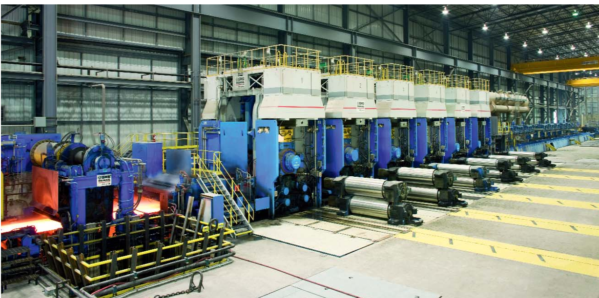
Fig. 9. CSP® mill at Severstal Columbus, USA.
