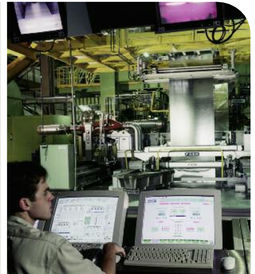
Control station in a continuous pickling plant
